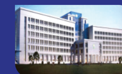
Governmental office building Rwanda
