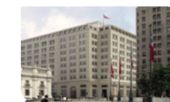
Governmental building Chile
